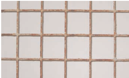
Hot Dipped Welded Mesh - Belmont Beach, NSW after 12 months
