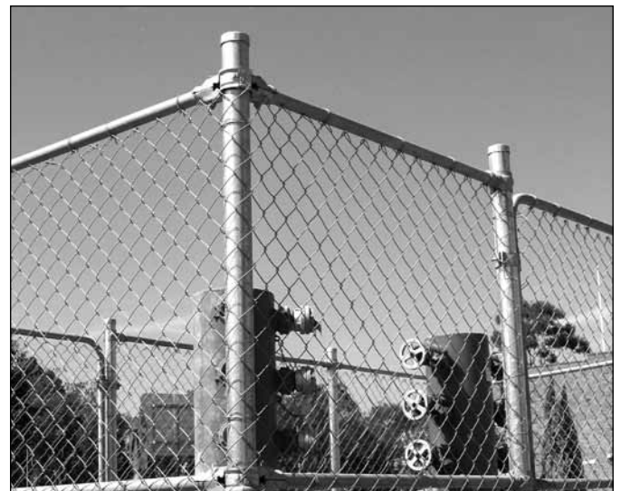
TYPICAL CHAINWIRE ENCLOSURE
