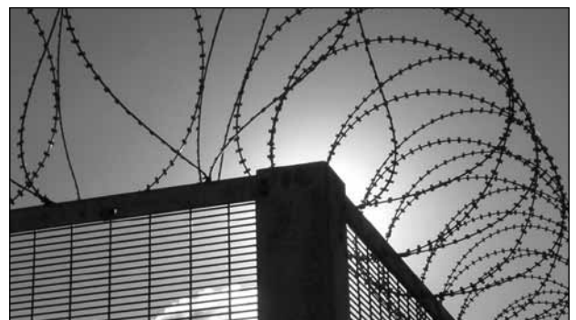
TOP RAIL WITH CONCERTINA RAZOR TAPE ATTACHMENT
