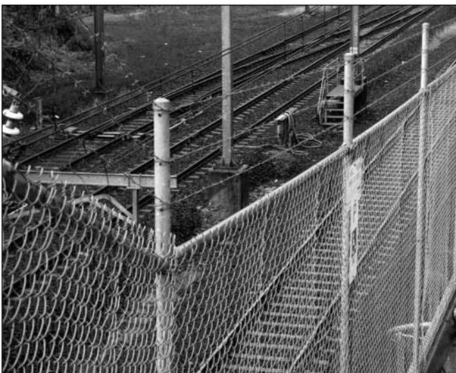
TYPICAL SECURITY CHAINWIRE FENCE APPLICATION
